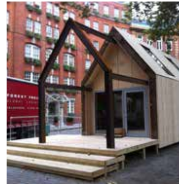
Circular Building, London 2016
