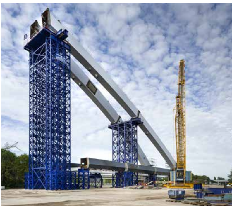
Montage Zandhazenbrug, Diemen
